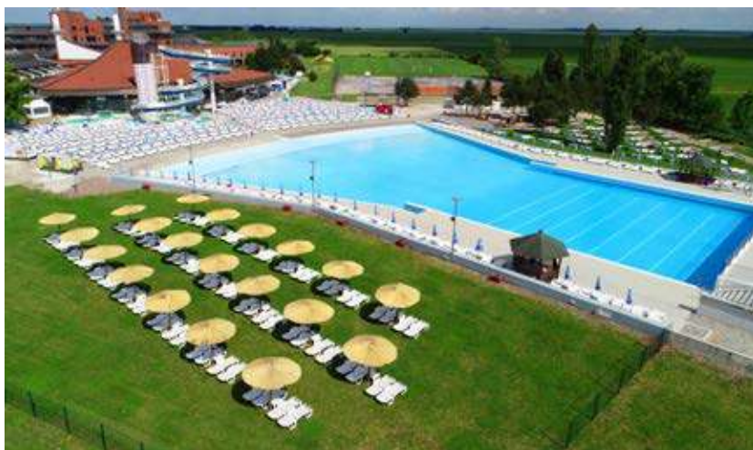
▲ THE SPA CENTER IN BIZOVAC
